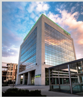
HQ Mansion of DKV, Spain
